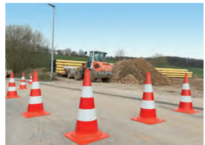
Construction site page 136
