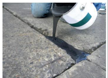
**RESTORE** Joint Repair is an extremely strong and durable two-component mixture with fast reactive binders for short curing times.
